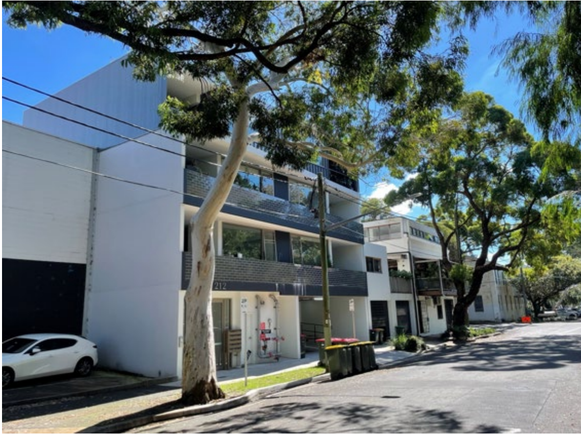
residential development to north - 169 Botany Road – viewed from Cope Street
