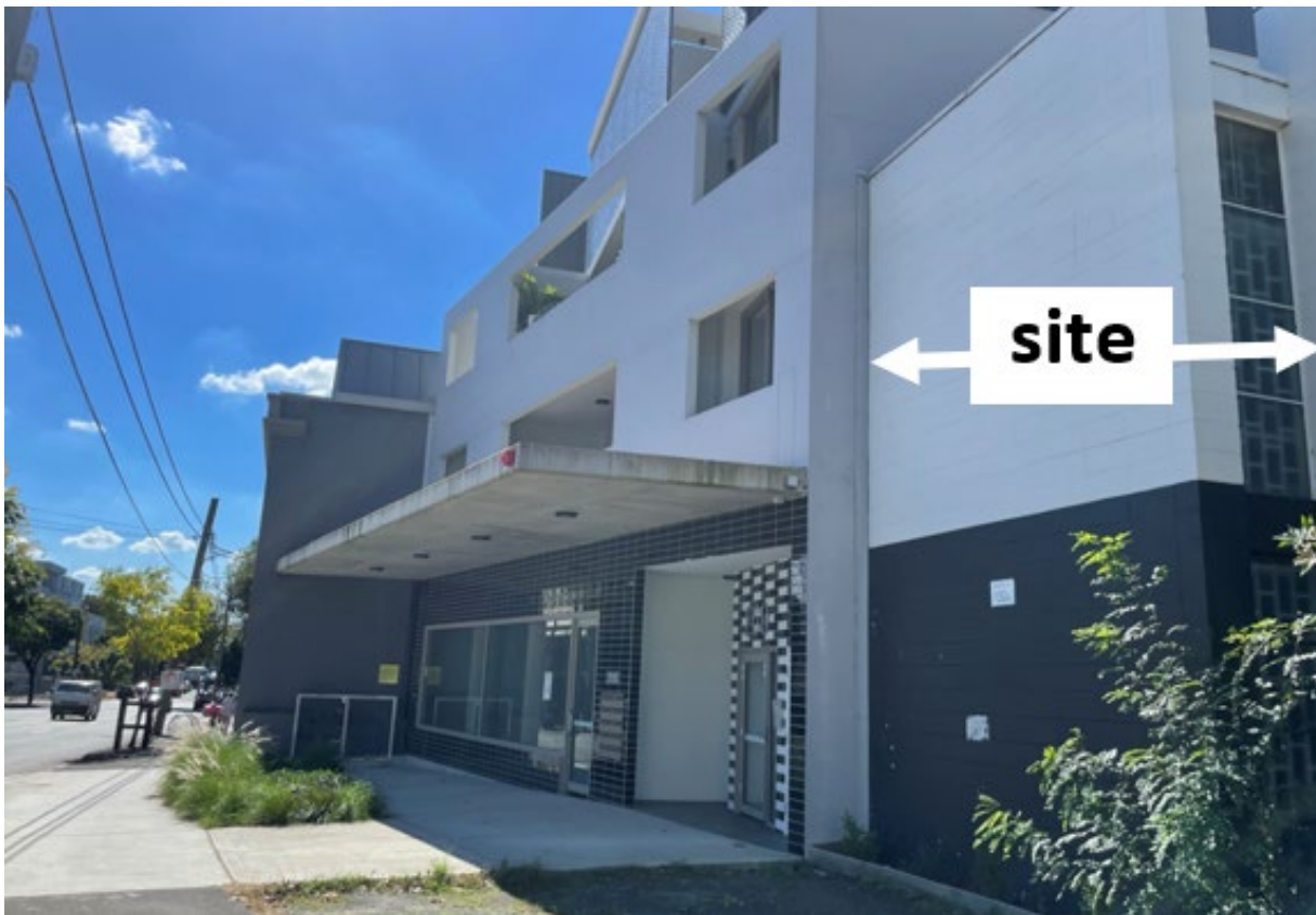
adjoining residential development to north - 169 Botany Road
